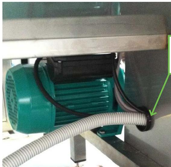
The above picture shows the main electrical cable entry point into the bike wash. Once you have run the cable and conduit to this point, leave another 1000mm for the termination inside the cabinet.
