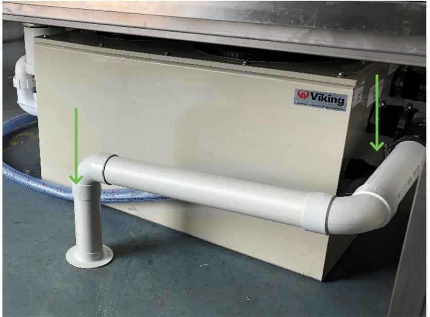
While the below picture shows the entrance point from the Bike Wash DBA (filtration system) to the Solvent & Oil Interceptor.
