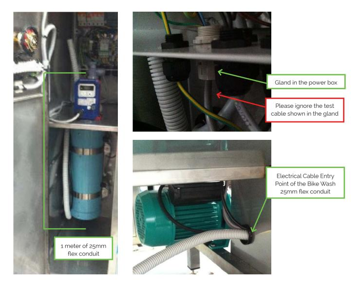
The above picture shows the main electrical cable entry point into the bike wash. Once you have run the cable and conduit to this point, leave another 1000mm for the termination inside the cabinet.
