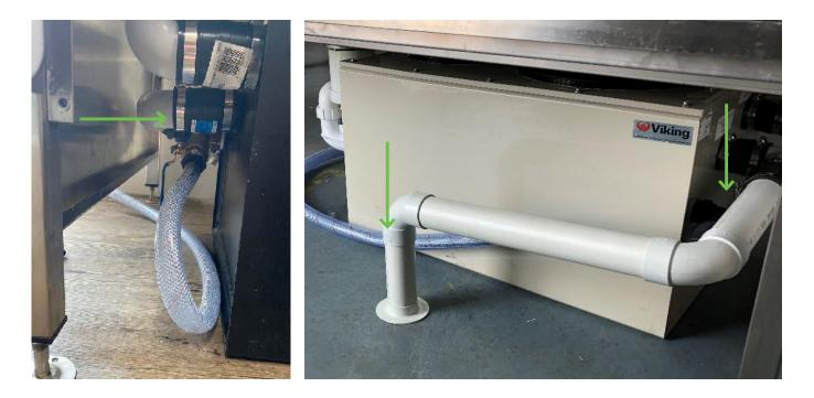
While the below picture shows the entrance point from the Bike Wash DBA (filtration system) to the Solvent & Oil Interceptor.
